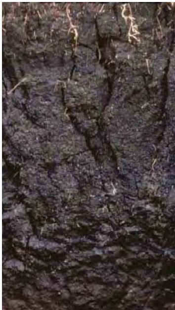
Soil cut showing the depth of cracking (about two feet) in an expansive soil
